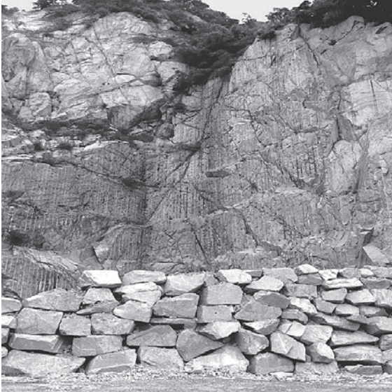
Figure 1. Mount Gokenzan, quarrying site of Aji stone.
